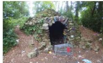
Item: Ice House Comments: Style and setting, intact but used as a rubbish dump and graffitied Category: 5 Item: Surrounding Woodland Comments: Original, shelter and character Category: 5
