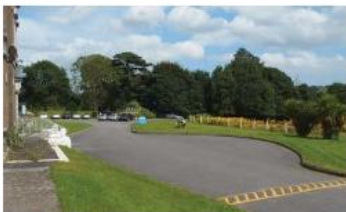
Item: Arrival Layout Comments: Curvature and scale Category: 4 Item: Concrete Kerbs and Tarmac Comments: Mid-1900's, replaced gravel Category: 1 Item: Cabbage Palms Comments: Frame to front door, period specific Category: 2
