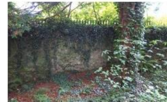
Item: Stone Boundary Wall Comments: Stone and plaster to 2.5m ht.; compromised at several locations Category: 5 Item: Woodland Understorey Comments: Clean, but only modest diversity Category: 3
